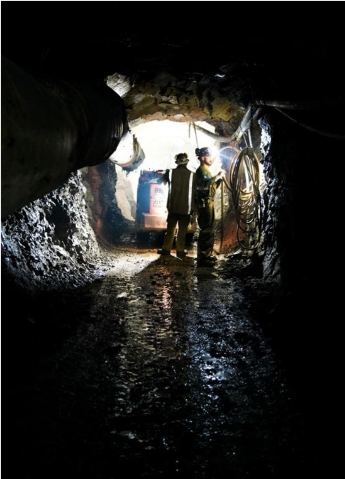
Figure: Crews advancing the crosscut to new underground drill station, August 25, 2026.
