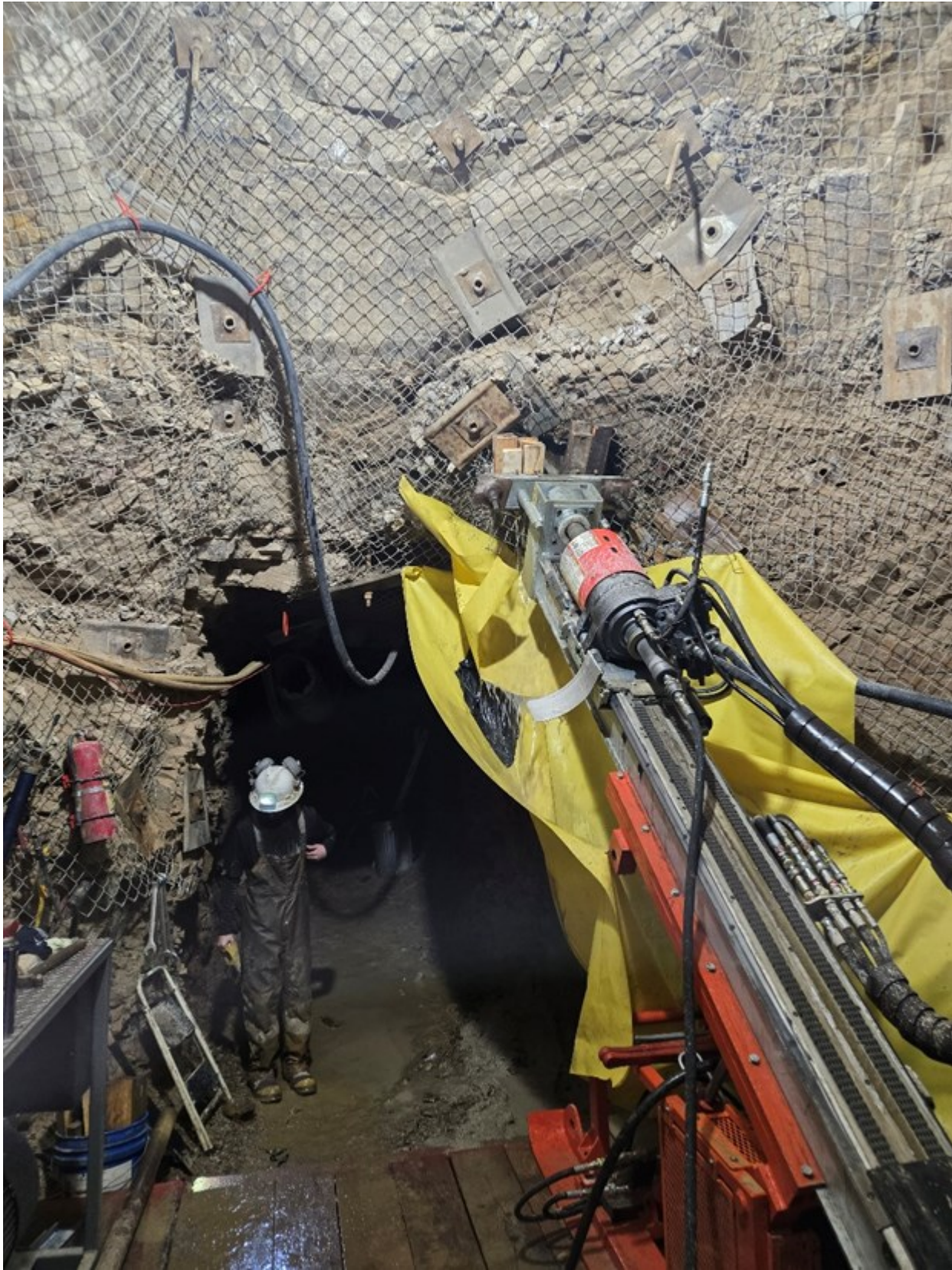
Figure 1: Drill Rig at the Zero Level
