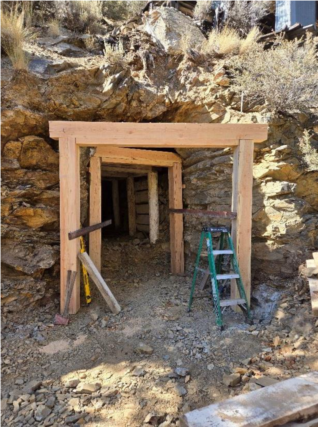
Photo 3 Rehabilitated portal entry-way to the Zero Level adit showing the first sets of timber installed.
