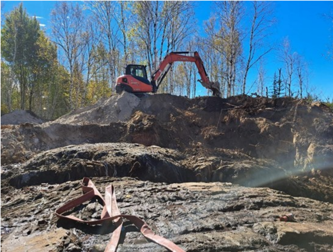
Excavator at Falcon Gold
