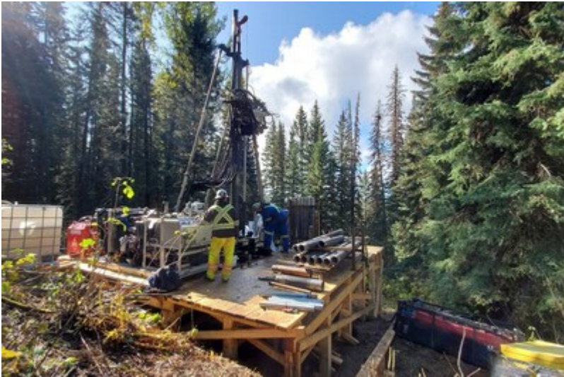
Image 1: Sonic Infrastructure Geotechnical Drilling Underway Within WSF Area (CNW Group/Defense Metals Corp.)
