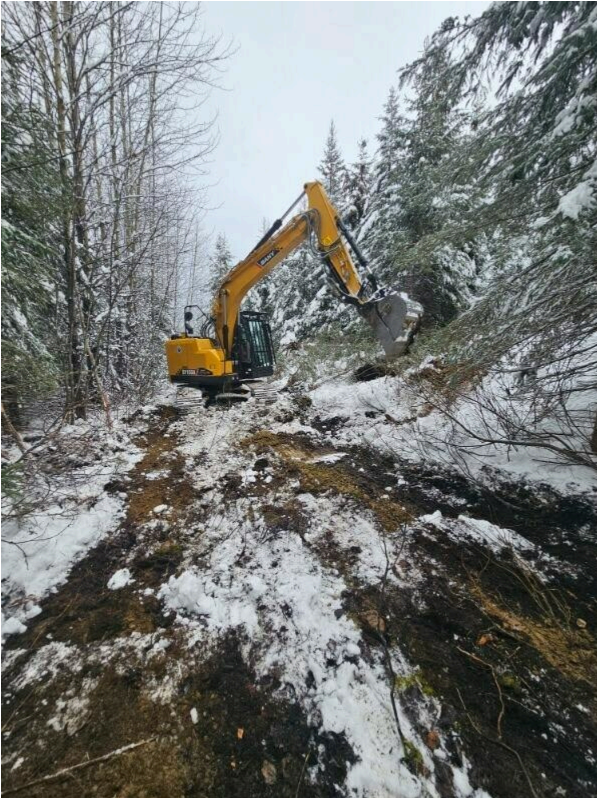
Image 3: Excavated Overburden Test Pits Underway in Tailings Study Area (CNW Group/Defense Metals Corp.)
