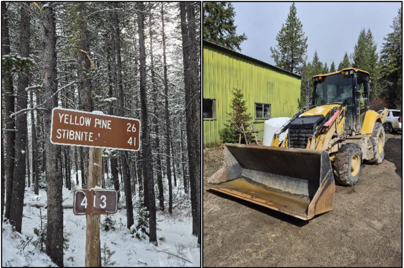
Figure 2: Access roadworks to Resolution's Horse Heaven Antimony-Tungsten-Gold-Silver Project.
