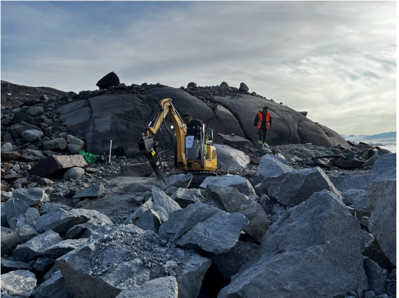
Blasted material being hammered into smaller fragments and loaded in bulk bags.
