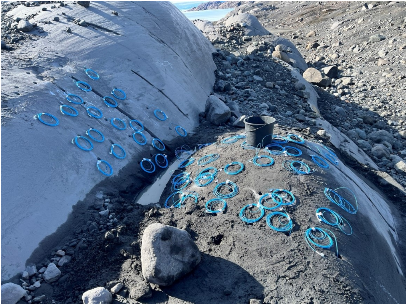
Holes loaded and ready for blasting at Skaergaard 2026.
