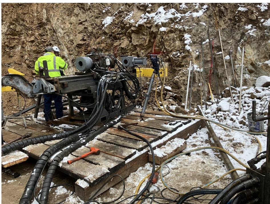
Contract Miner at Face at Washington Mine
