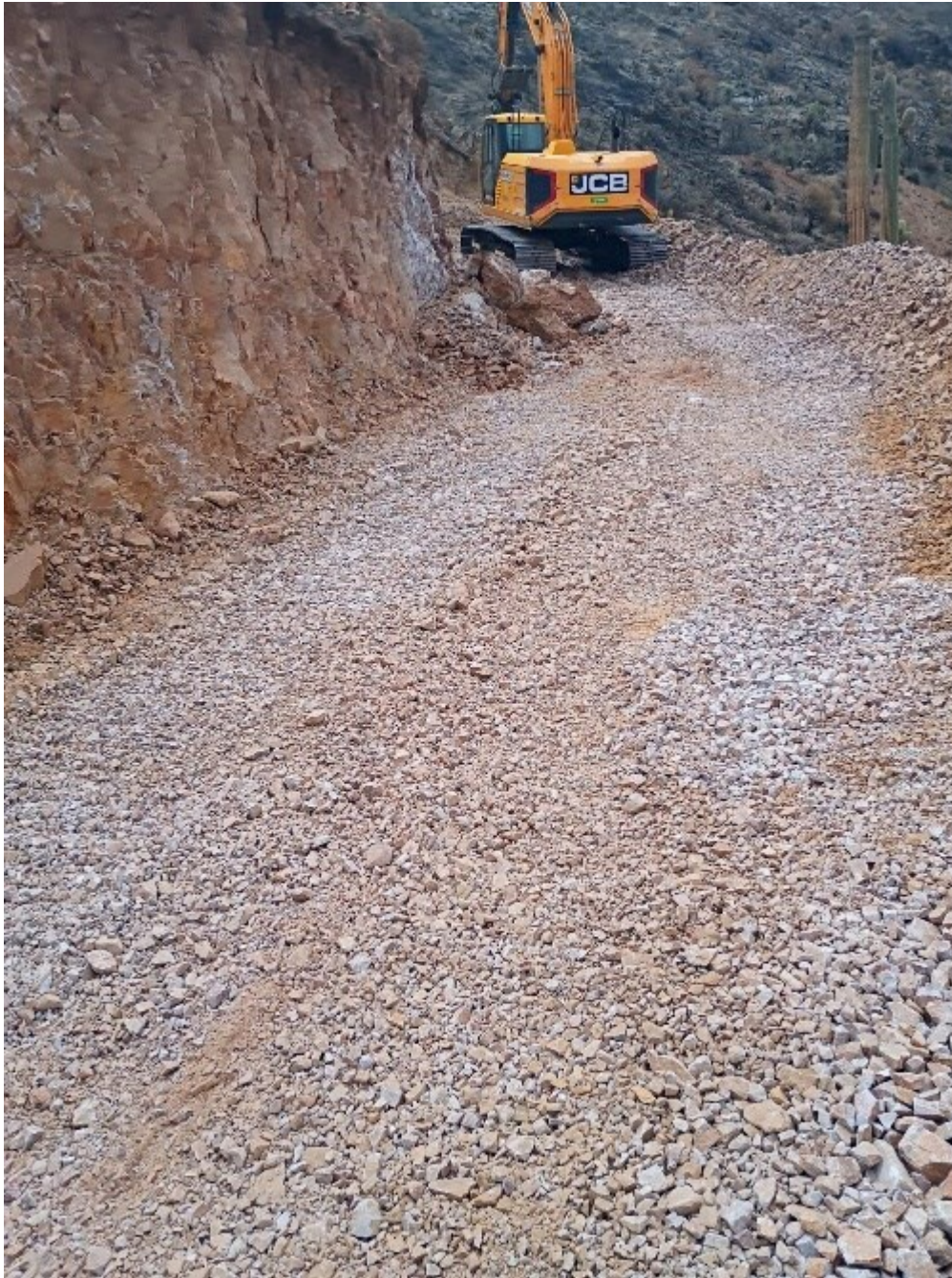
New Road Being Completed to Gold Queen Mine
