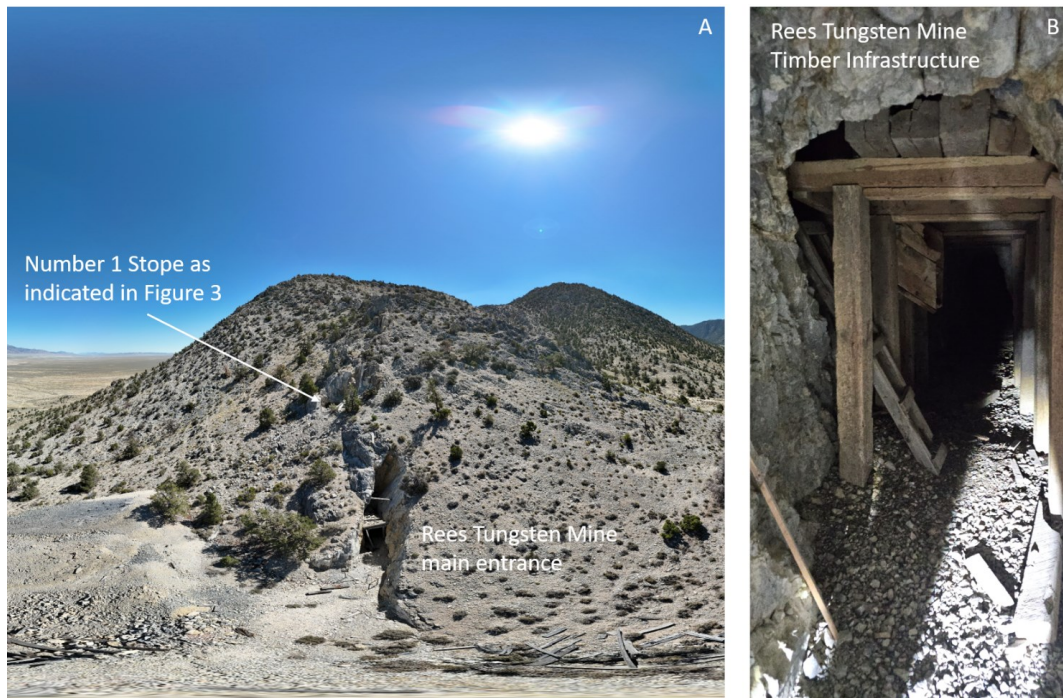
Figure 6 Aerial photo of Rees Mine (A) with example of timber infrastructure and chute remaining in the main adit (B).
