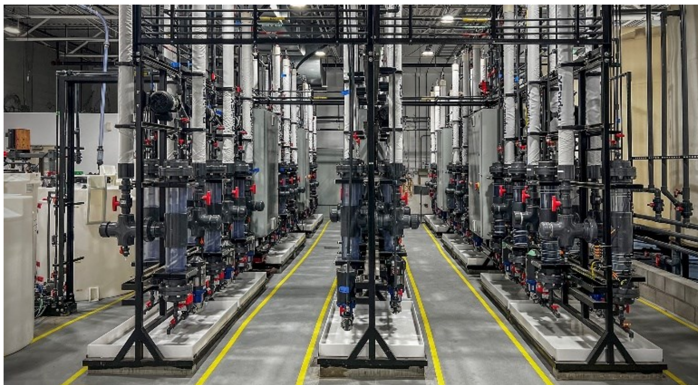
Figure 1 – 52-Stage RapidSX™ Demo Plant
