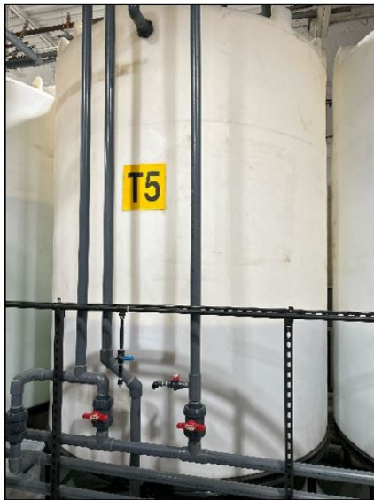
Figure 1: Thousands of liters of separated rare earth chloride products: T5 Raffinate (La, Ce, Pr, Nd, Sm, Eu, Gd, Tb, Dy), T2 Strip One Liquor (Ho, Y, Er, Tm, Yb) and T3 Strip Two Liquor (Yb, Lu) – each tank has a 17,400 liter capacity.
