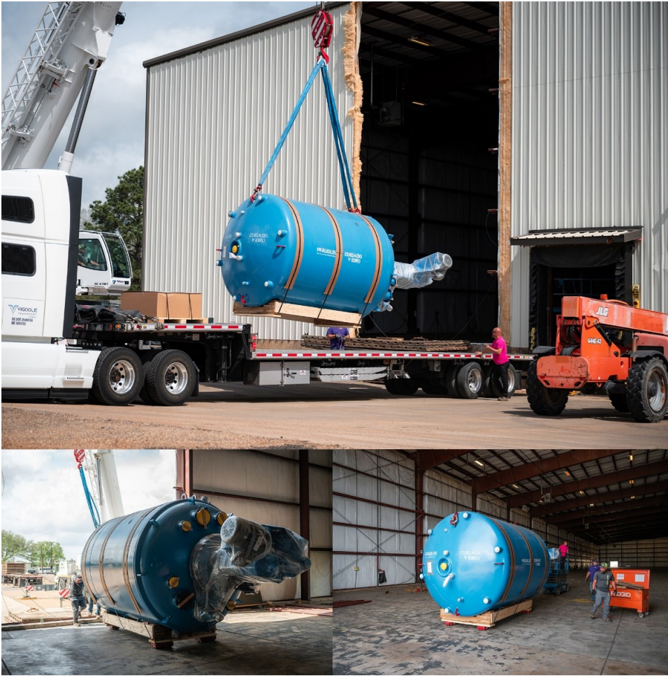
Figure 1 – A 4,000 Gallon Pfaulder Leaching Reactor Arriving at the Louisiana SMC
