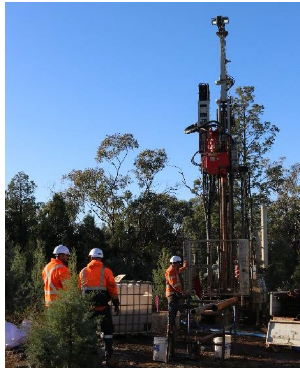
Core drilling and sampling at the Dubbo Project, part of the RE Options Assessment work.
