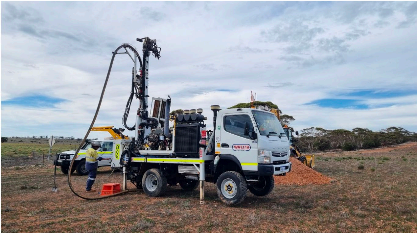
Rig on first location
