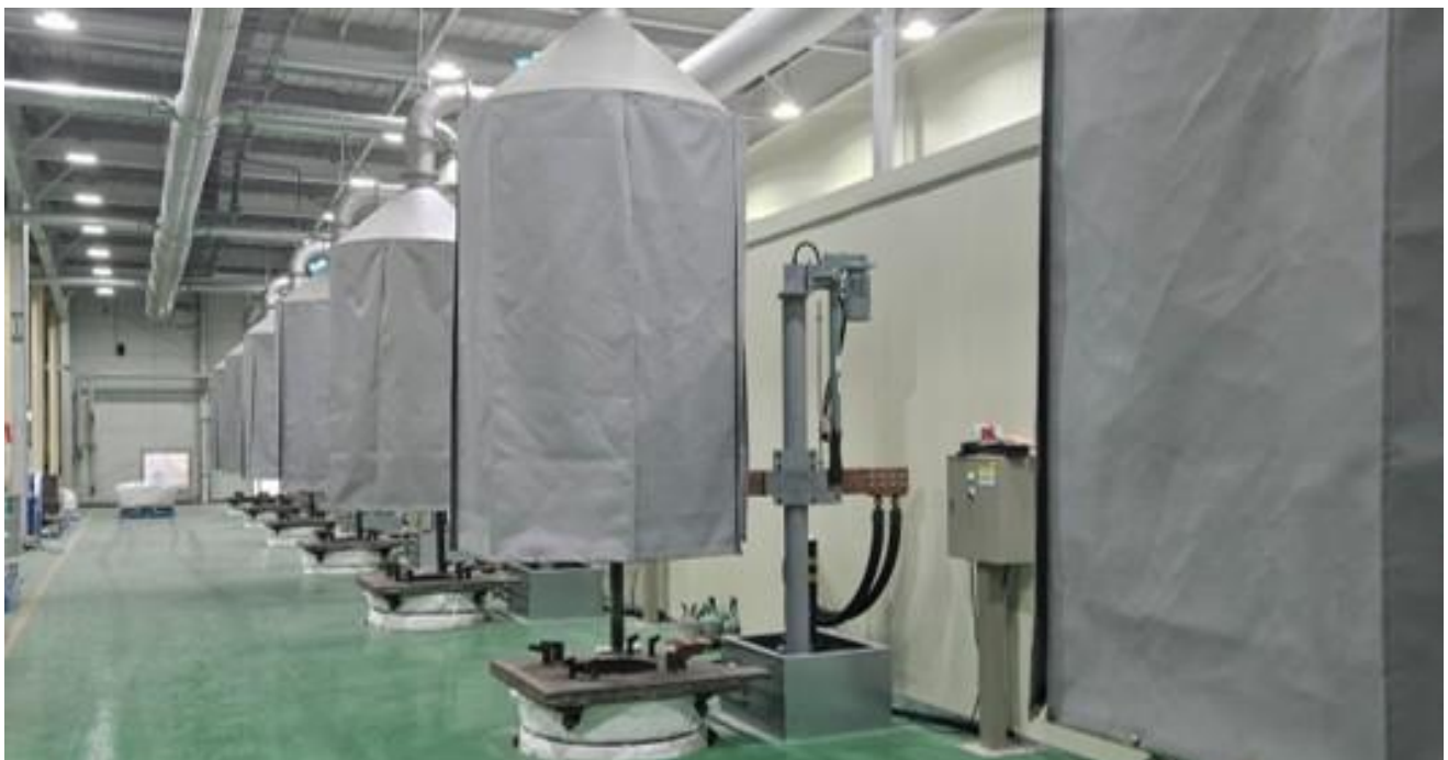
The new furnaces installed at the KMP will support the facility's ramp-up to a nameplate production capacity of 3,600tpa of alloy.
